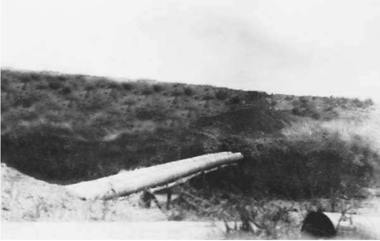
13. Double 20-inch pipeline bridge at camp 25.
