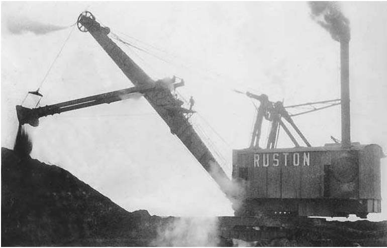
6. The big shovel at work at camp 1060.
